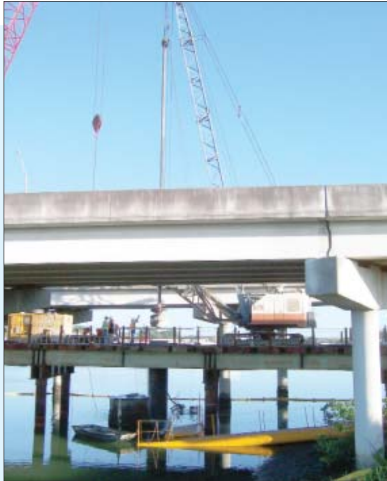
Remediation work being done on shafts out in the Palm River.
