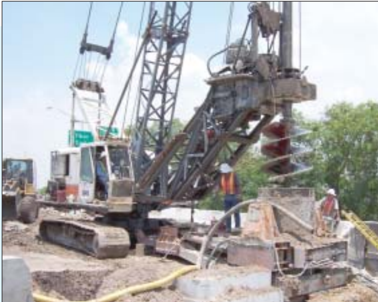
BECK-manufactured hydraulic crane attachment mounted on a Northwest 5045 working on remediation shafts with no overhead obstructions.
