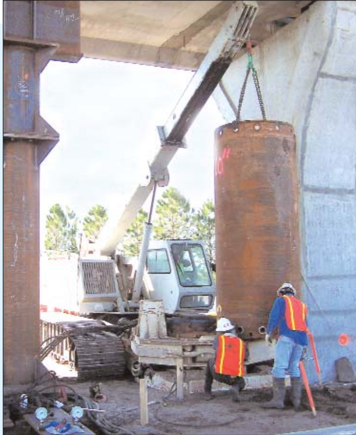
BECK-modified casing oscillator used to advance casings down to the limestone.
