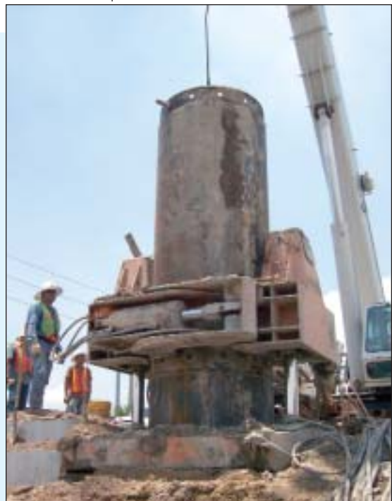
Casing being extracted after concrete placement.
